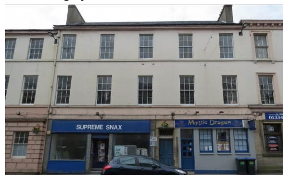
West Wing after dormer windows removed:
