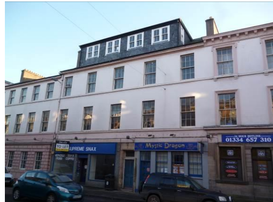
West Wing before works started:
