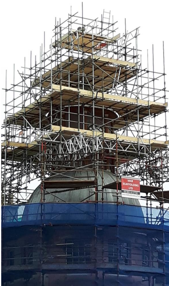
The extensive scaffolding to the dome and clock tower:
